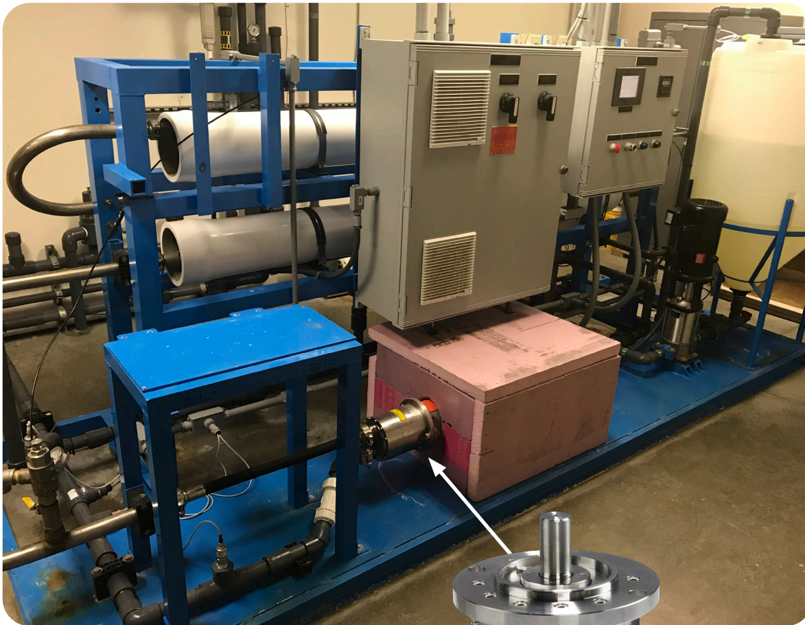
↑ The APP 7.2, installed on a remote island in Washington's San Juan Islands, ran for 11 years with zero maintenance.
