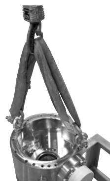
30. Mount 2 lifting eyes across from each other in the stator housing to equal the weight and use a lifting strap to lift the stator housing.
